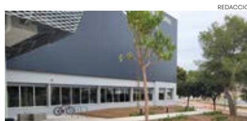
Accessos reformats al CEM Can Roca
